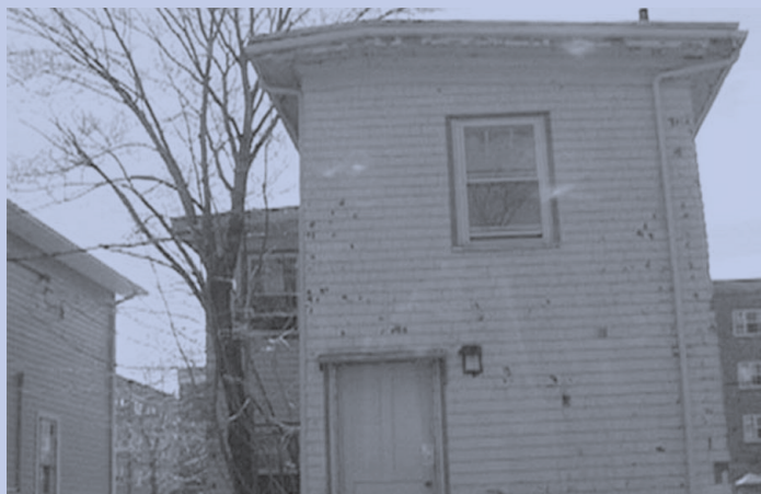
HALIFAX. Project Class house, back view. Photo David Askevold, 2005.
